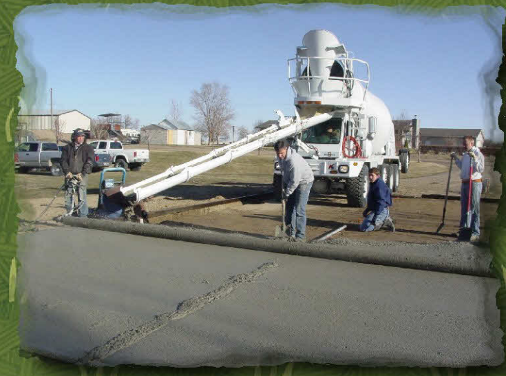
Pouring the massive 24' X 50' pad was the pavilion's first challenge
